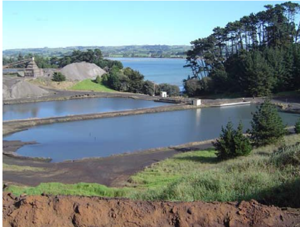
Figure 4: Northern side Storm water Ponds, NZ Steel
