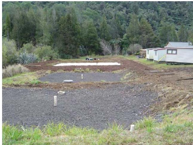
Figure 3: Waipoua Forest Filter beds
