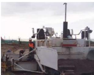
and the Illawarra Highway Albion Park Rail. The runways, taxiways and hardstand areas were completed with selection of Slag Base RBU800 – 80/20 material (of the same type used for the base of the Sydney International Airport third runway project dating back to 1993) in 300mm layers of up to 750mm in thickness.
