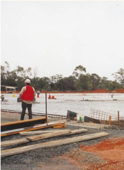
**Cobar is the only place in Australia where crushed copper rock slag is regularly used as an aggregate for concrete**
