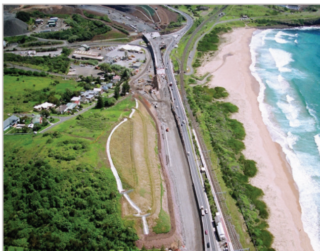
Figure 5.3 - Aerial view of completed project.
