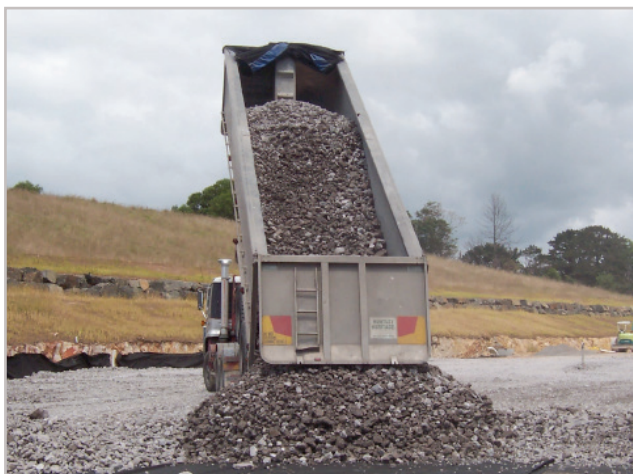
Figure 5.2 - Truck unloading slag material at site.
