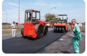
Through discussions with one of the consulting engineers, it was evident that the current natural aggregate at one particular location was causing problems with the asphalt quality. The asphalt was deforming at a very early stage and the binder was stripping from the asphalt due to poor quality fines. It soon became apparent that the properties that steel slag had to offer could possibly present a solution to these problems. CONT PG 5
