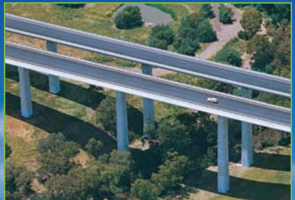
ABOVE: EJ Whitten Bridge
