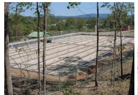
Vertical filter bed at Rocks Riverside Park Brisbane Dec 2004 when the reeds were newly planted.
