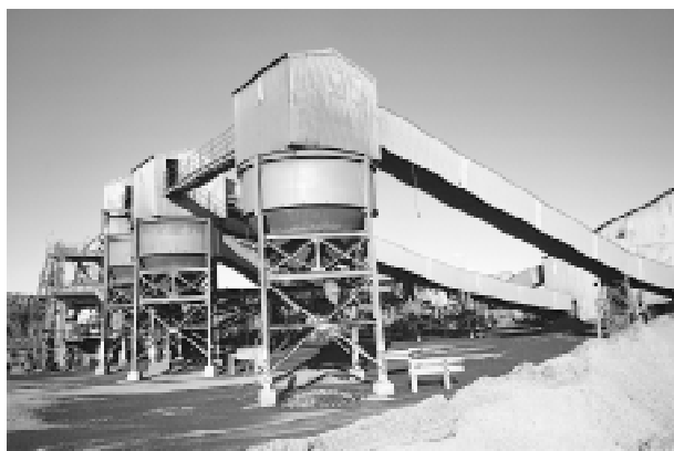
Steel Furnace Slag Processing Plant, Port Kembla NSW.
