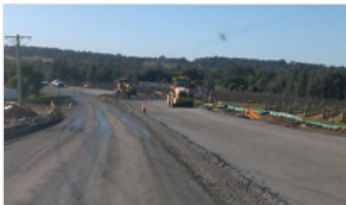
Figure 1 - Longitudinal construction jointing.
