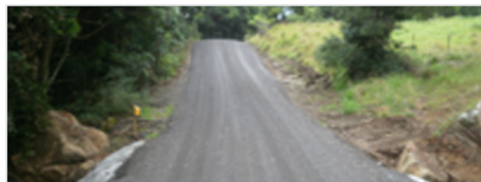
Figure 3 - SFS road base used at Misty Lane, Jamberoo.
