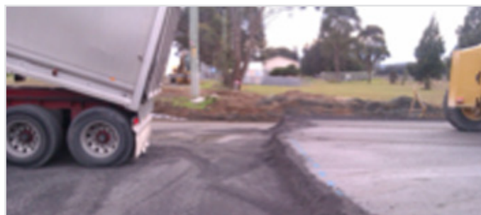
Figure 2 - Transverse construction joint.
