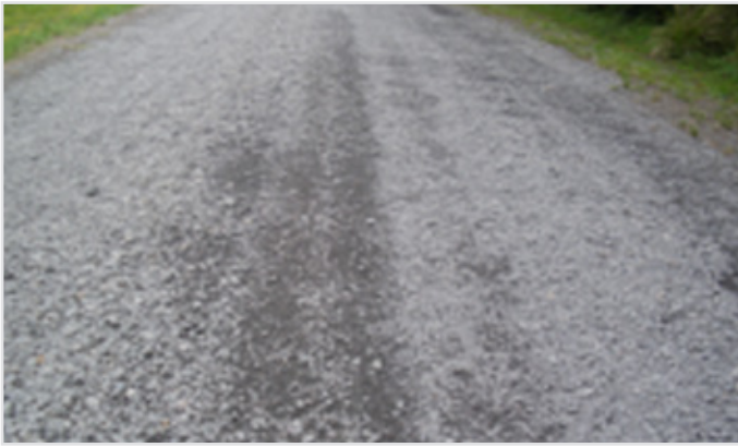
Figure 4 - Close-up of SFS road base.
